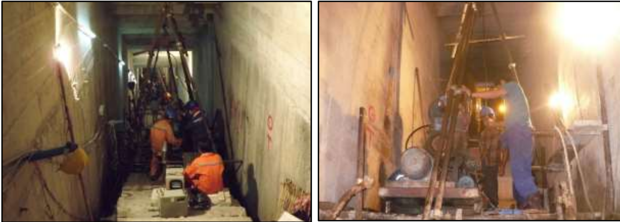
Figure (16) Curtain grouting inside the foundation gallery at UPL dam
